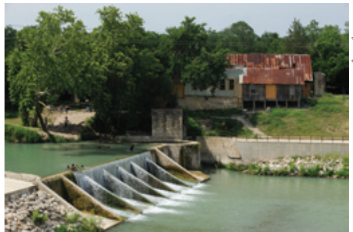
Dam in the San Marcos River at Zedler Mill, Caldwell County.
